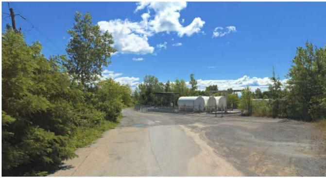
IMAGE 2: END OF SUNSET DRIVE ASPHALT PAVEMENT & TRANSITION TO AGGREGATE PAVING
