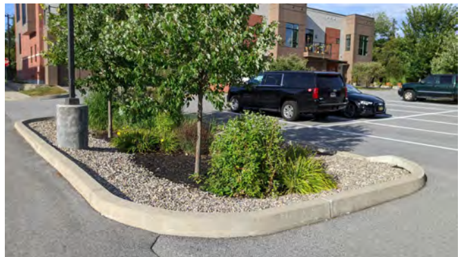
Figure 24. Stormwater retention in a parking island.
