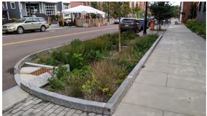
Figure 23. Stormwater retention with raingarden.
