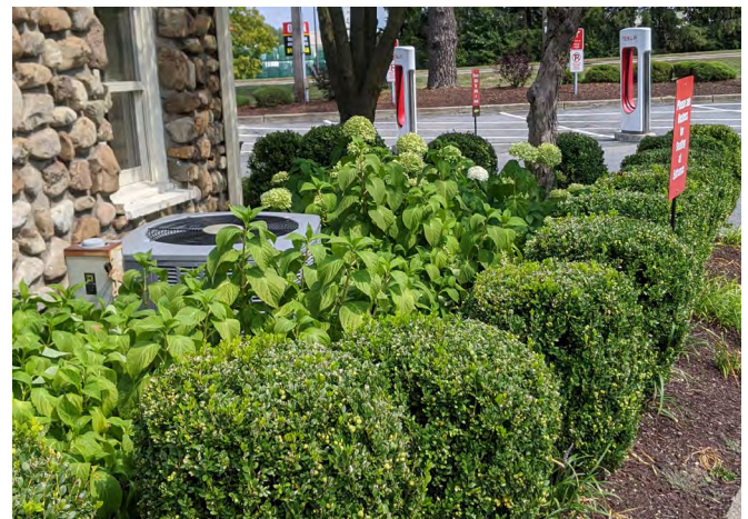
Figure 31. Screening of mechanical equipment using landscaping.
